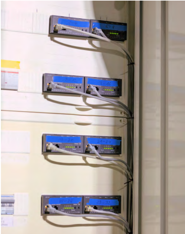
Reliable control: Expert Net Control 2302 used eight times in the new SoundLab Photo: Fohhn Audio AG
